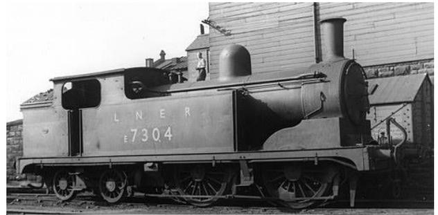
(LNER Class G5) 0 - 4 - 4 Passenger Tank Locomotive
